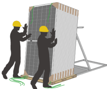
7) Cut off the remaining packing belts so that the modules rest on the auxiliary tool.
